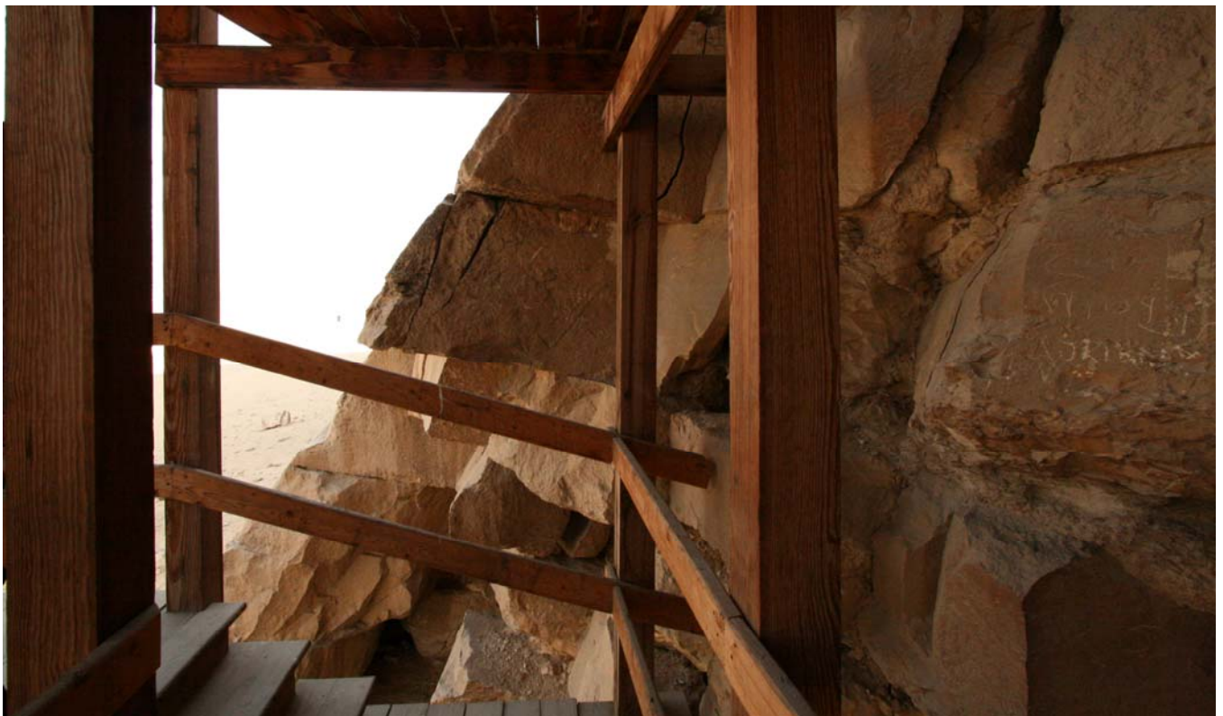
In the dismantled area by the entrance on the north face of the "Bent Pyramid" of Snefru (Snof-Ra) at Dashur we can clearly see that the blocks were laid tilted at a slight angle towards the centre of the pyramid.
